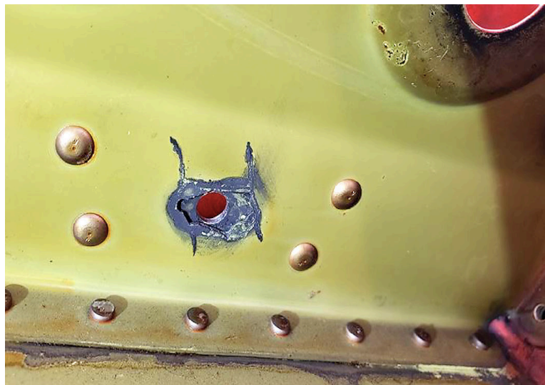
Right: Pilatus PC-12. Underside of rudder rib 6 with missing anchor nut.
