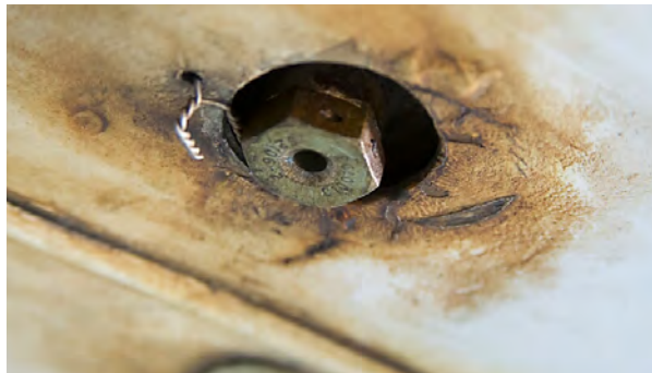
Left: During inspection pay special attention to attaching hardware, such as bolts or pins.
