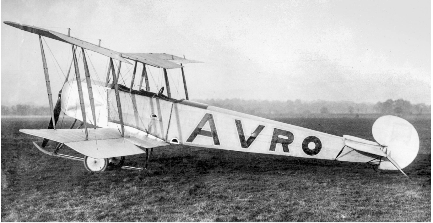
Above: Avro 504 prototype after modification with conventional ailerons.
