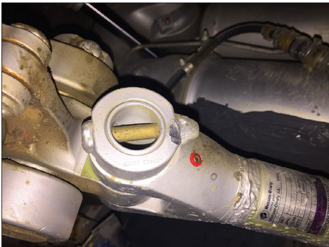
ATR42 320-Incorrectly installed collar which shows evidence of contact with link unit.
