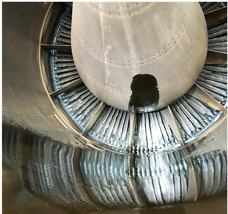
Above: General Electric. View of engine tail cone after nozzle failure.
