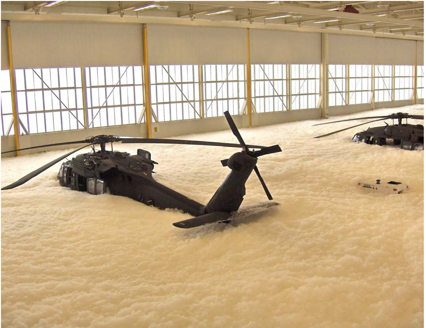
Above: The most common damage seen in the aftermath of a foam discharge event relates to brake assemblies, avionics and engines.
