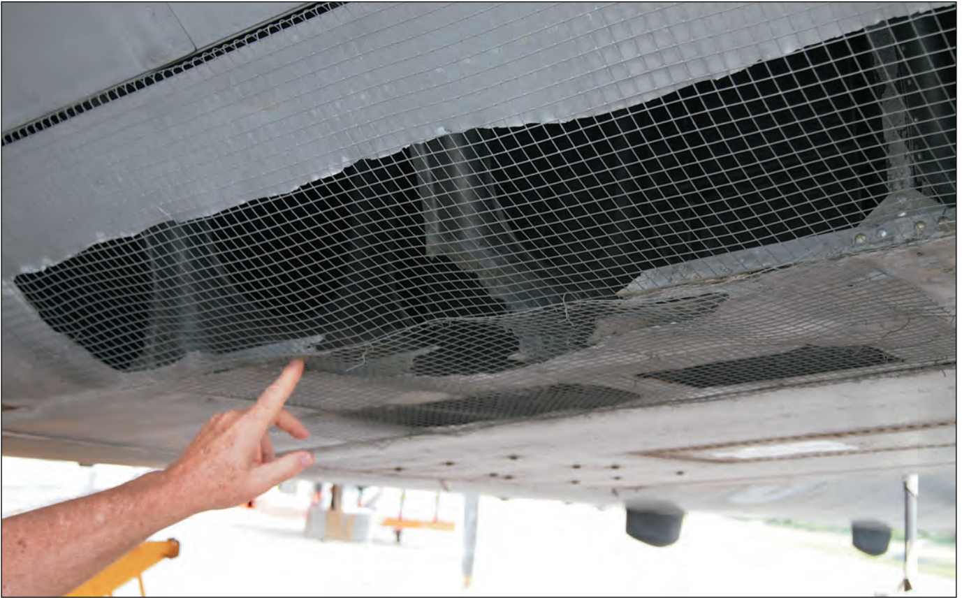
Bill Tate points out corrosion caused by bird droppings.
